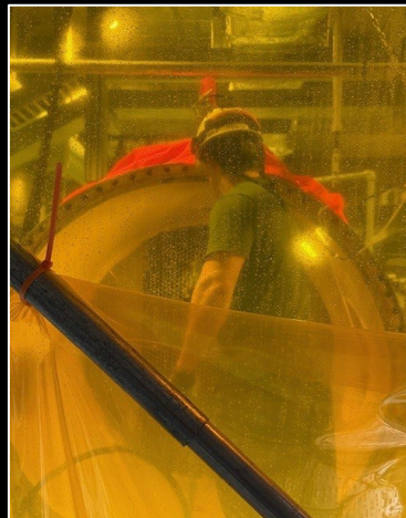
Right: Jessie Padgett hydrolazing ACCW; Jessie Padgett hydrolazing 3C FWH
