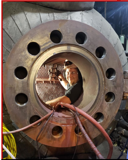
Left: Andy Mills cleans the Turbine Lube HX at Brunner Below: Jeremy Bajenski probe handles at Montour Right: Steve "Banjo" Joiner & Dan Perak inspect the Glam Steam at Harris
