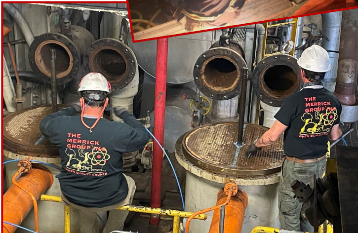
Below: Dan Corcoran & Wayne Chonko clean the Main Turbine Lube Oil Coolers at Brunner Island
