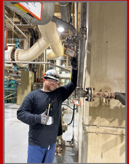
McGuire HX Jake Young finding water source for Condensate Coolers cleaning
