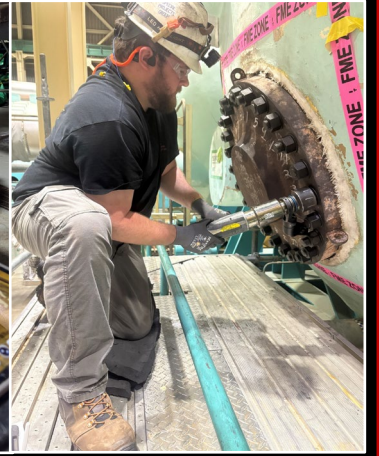
Luke Gergely torquing manway at Catawba
